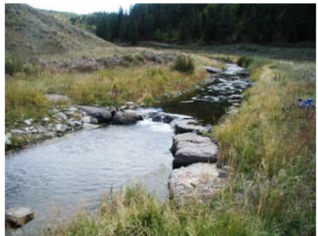
Figure TS14G-9 A J-hook grade control structure
